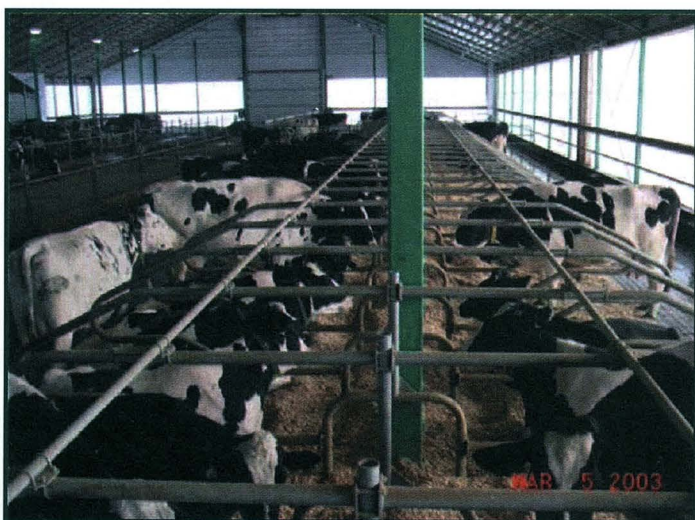
Figure 5. Forward open space facilitates straight standing and lying in stalls. The forward open space in these 18-foot stalls also permits front lunging, heat dispersion through cow separation, and avoidance of dominant/subordinate behavior.
