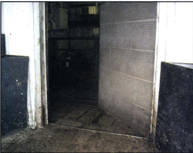
Photo 9. Door guides at plant entrance.
