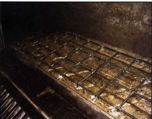
Photo 14. Welded grating on stun box floor.
