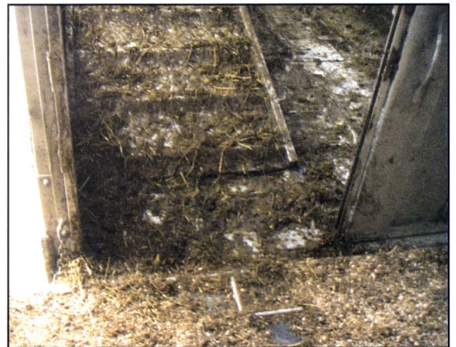
Photo 6. Steel grating on landing to improve footing.
