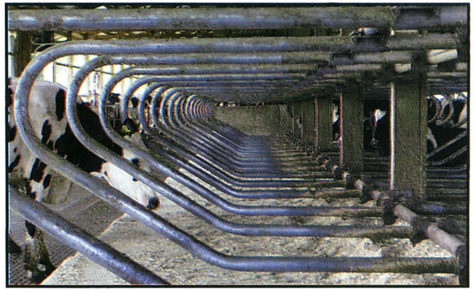
Figure 11. These dividers are mounted on a horizontal rail that intrudes into the bob-zone in these 7.5 ft (2.3 m) stalls. The lower rail of the divider reaches 10 inches (25 cm) above the mattress, which allows side lunging.
