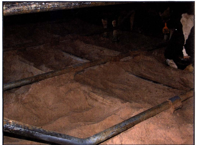
Figure 3. A transverse mounting pipe is retained in this stall, but mounted below the bedded surface in a sand free stall. The bedding has been moved to show the bar and the right-angle mounting bracket.
