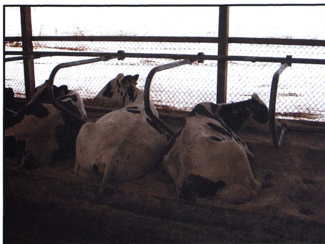
Figure 1. Remodeled sand stalls in a mature cow free stall pen. The stalls were widened from 45 inches to 50 inches (114 cm to 127 cm) wide on center.
