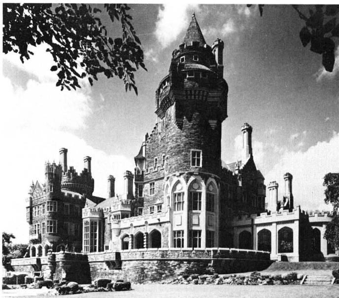
Casa Loma — Toronto's 98 room castle.
