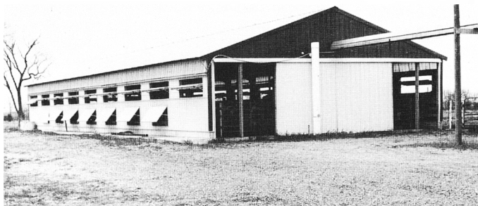
Figure 19. Totally slatted floor young stock building 40' x 108'. Wall height is 11 feet. Upper row of ventilation doors initially built did not permit sufficient summer air movement for uniform environmental conditions. Lower doors 6' 8" x 3' were added on both sides and have corrected the problem. Continuous, unobstructed ridge opening is 10 inches wide. Roof is built of prefabricated insulated panels smooth on the underside to prevent condensation in winter and heat gain in summer. Inside temperature in summer approximates that of the outside.
