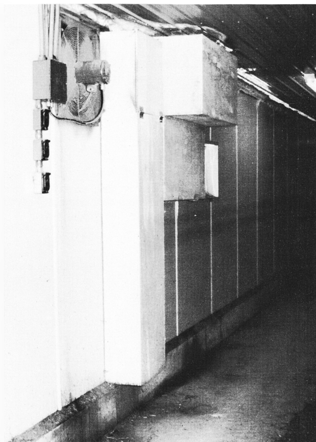
Figure 4. A close view of one group of fans in the barn shown in figures 1 and 2. The duct is built around a minimum capacity fan, which operated continuously during the winter of 1981-82 when outside temperatures fell to -40° or lower. The spring and fall fan at the left is thermostatically controlled. What appears to be a box at the right is an insulated, removable cover for a fan that operates only in summer. This prevents air leakage through and ice formation on the shutters in winter.
