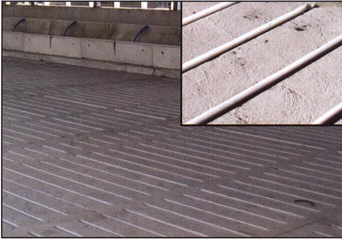
Figure 5. Study pen with slatted concrete floors and close-up image of concrete flooring.
