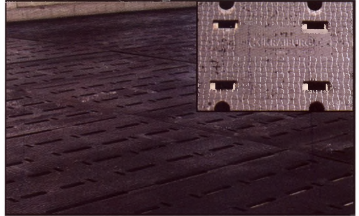
Figure 3. Study pen with Kraiburg™ rubber mats installed over slatted concrete floors and close-up image of mat.
